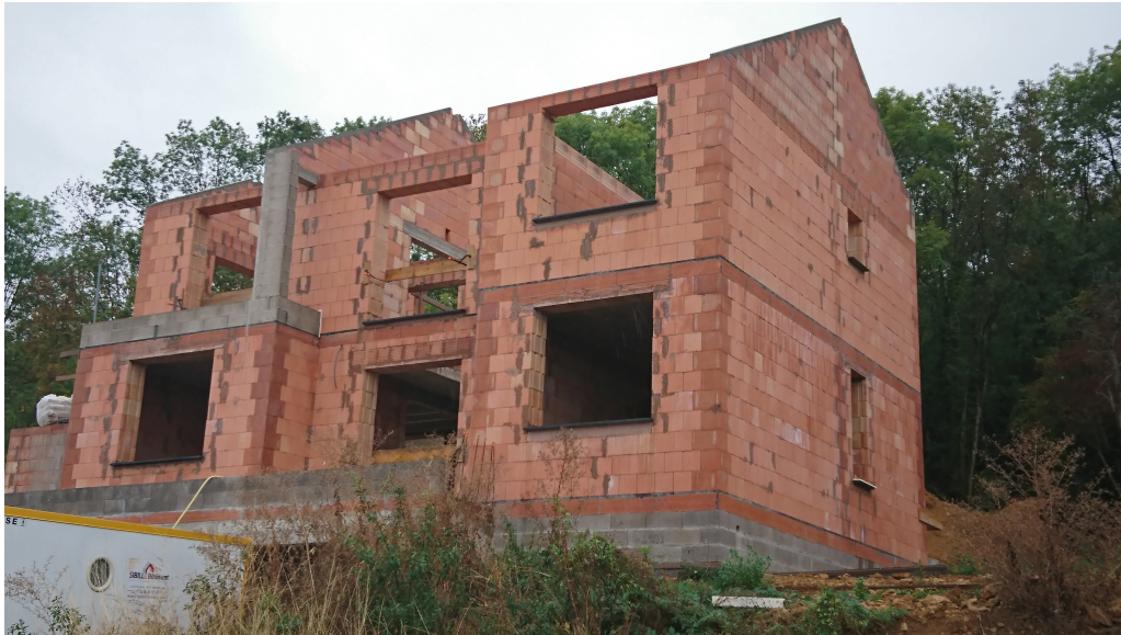
Figure 1.8. Construction des murs, linteaux, pignons
